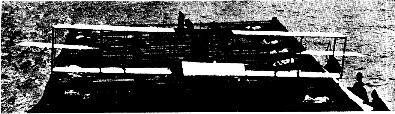
PRIMITIVE ARRESTING GEAR comprised of 22 taut ropes weighted by 50-pound sandbags were strung four inches off the deck of USS Pennsylvania for Eugene Ely's historic landing. Plane had three hooks beneath it to catch ropes. DFC was awarded Ely posthumously in 1933.
